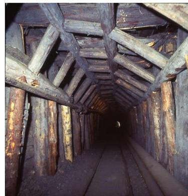
The majority of the tunnels in the mine are supported by wooden beams
